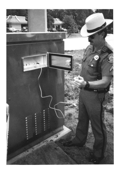
When under manual control the controller will stop timing the phase, allowing it to remain in that phase until the push-button on the manual control cord is activated. When the push button is activated, the controller will proceed to the next phase. If the push-button is not activated the controller will remain in the current phase indefinitely.
