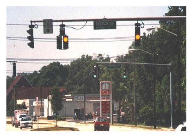
This allows vehicles to clear all the way through the intersection instead of getting caught in the middle between the two side street approaches. The duration of the delay between the first set of heads turning yellow and the second set of heads turning yellow depends on the value that is programmed into the controller as the independent overlap's green interval.
